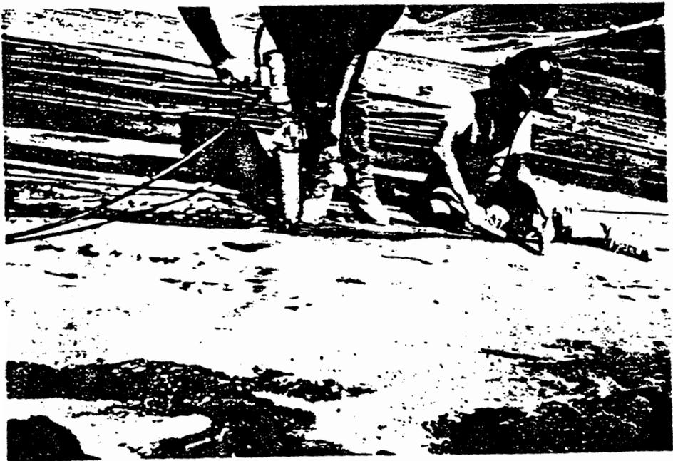
Figure 8. Field seaming geomembrane using a hot-extruded fillet weld. Worker at right is cleaning and wire brushing overlapped area to be seamed.
