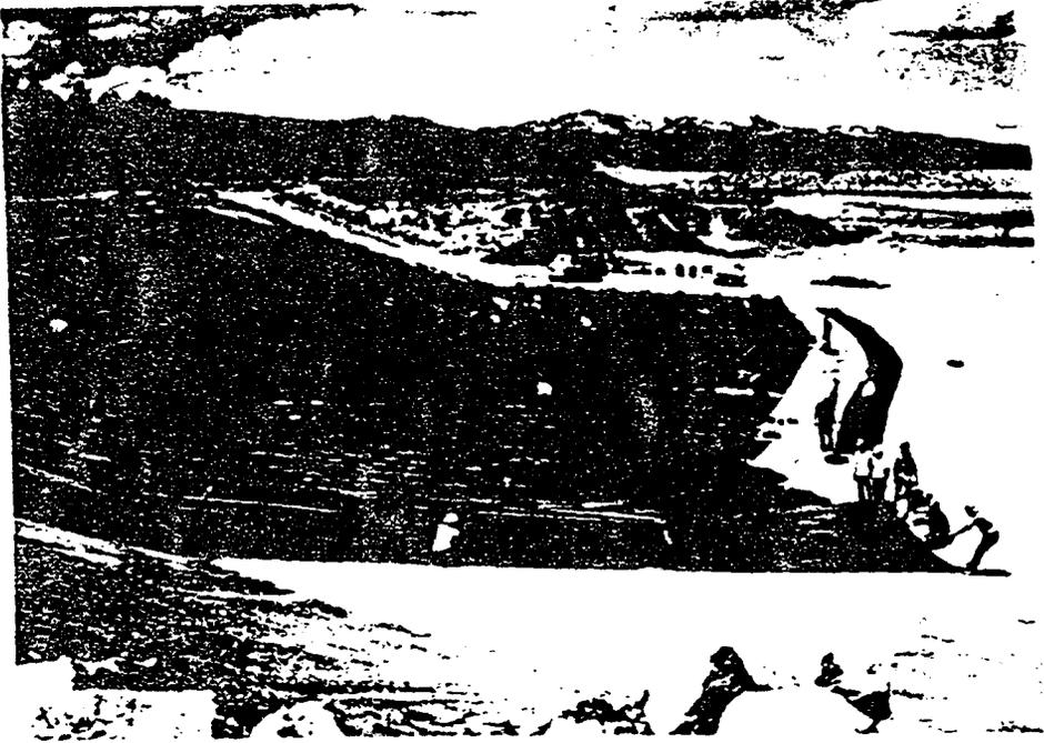
Figure 2. Installation of geomembrane on reservoir side slopes.
