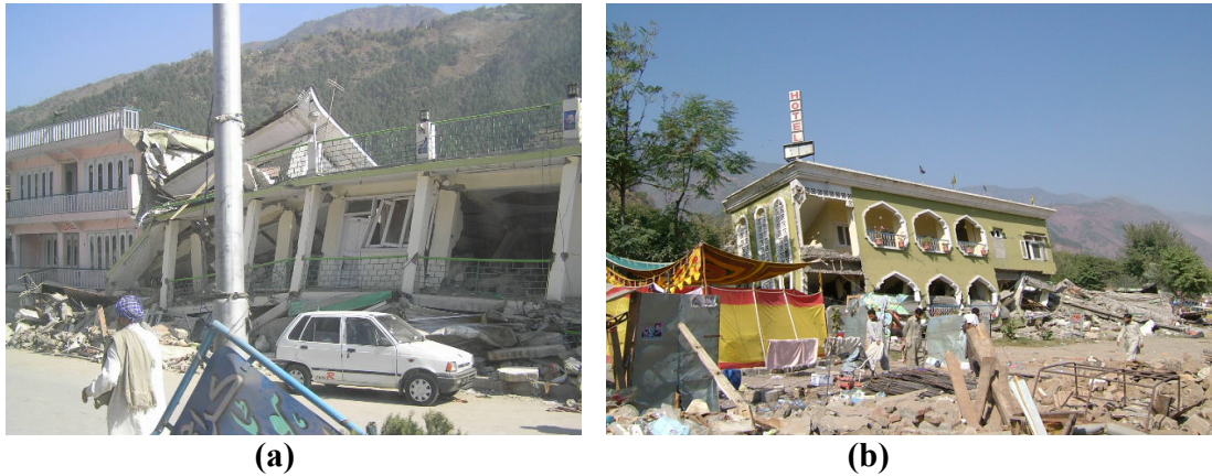
Figure 5: (a) Collapse of masonry building in Muzaffrabad due to settlement (b) Collapse of masonry building in Balakot due to settlement
